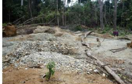
Spoil heap derived from washing of shallow surface lateritised saprolite
