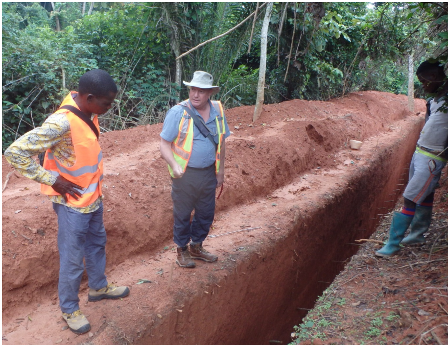
Trenching at Ziatoyah discovery, Nimba Project
